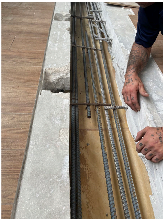
Picture 1: Excavation at Unit 108
